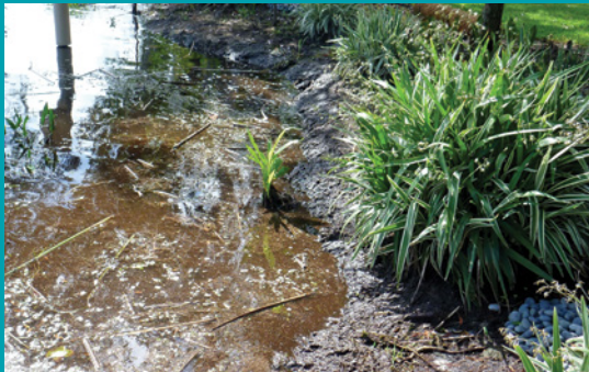
Shoreline erosion due to wave action.
